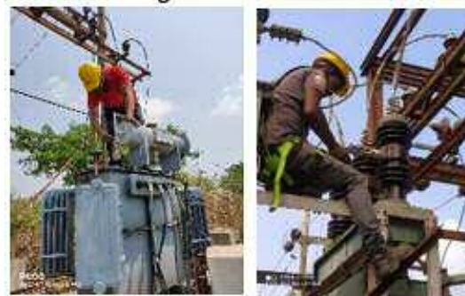
Maintenance of DT & Sub-station Equipment
