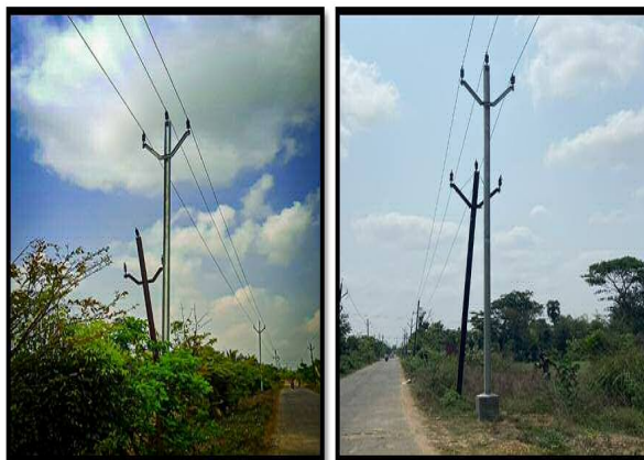
Photographs 11-1: Increasing Vertical Clearance
