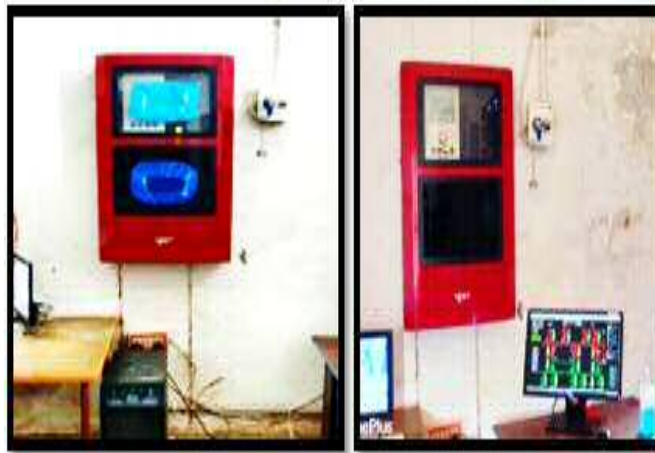
Photographs 11-6 : SCADA Enabled FDS
