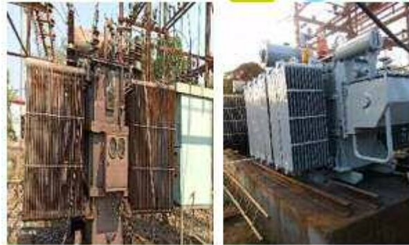
Overhauling of Power Transformer
