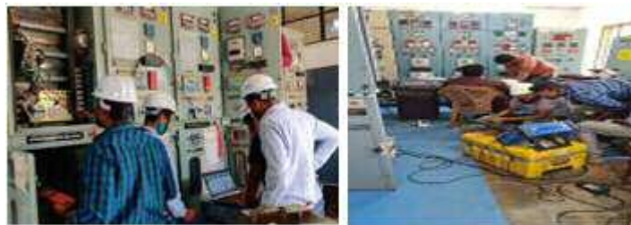
Technical Audit of 33/11 KV Sub-stations
