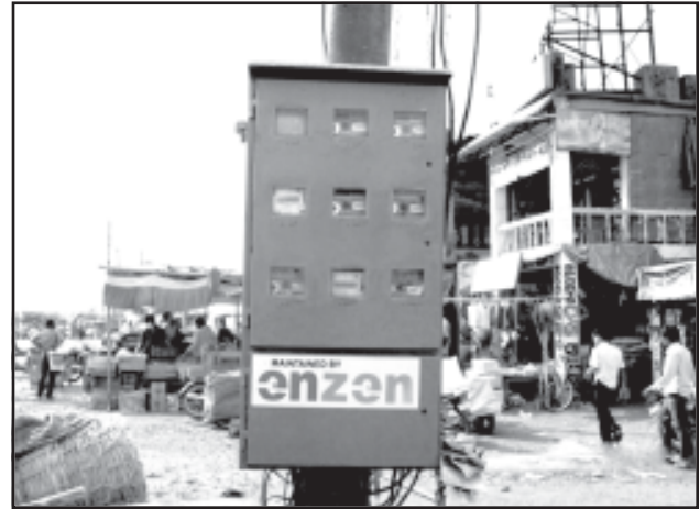
After Pole top Metering
