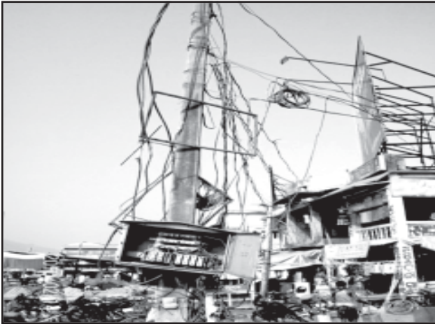
Pole condition Before Pole Top Metering
