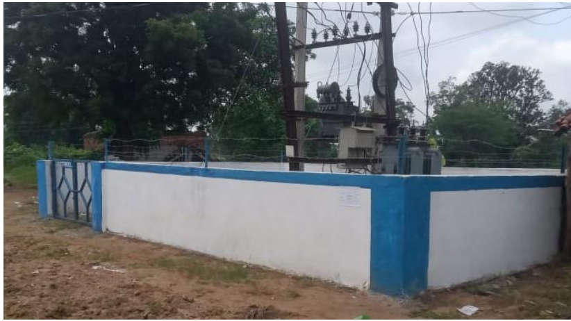
DTR fencing at Sunalarambha, Thuapali, BED under Bargarh Circle
