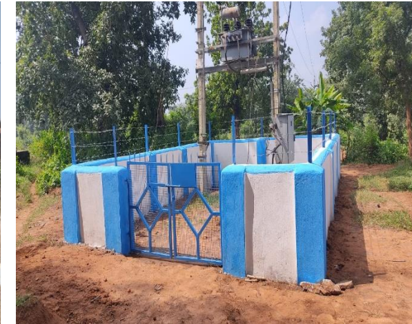
DTR fencing at Dhatukpada, BNED, under Sambalpur Circle
