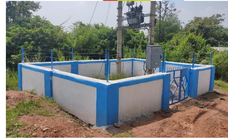
DTR fencing at Betjharan 1, BNED, under Sambalpur Circle
