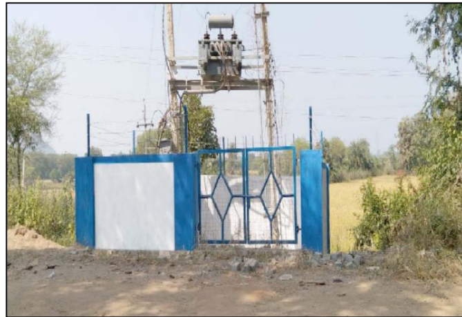
DTR fencing at Badamaheswar, NED, Under Kalahandi Circle
