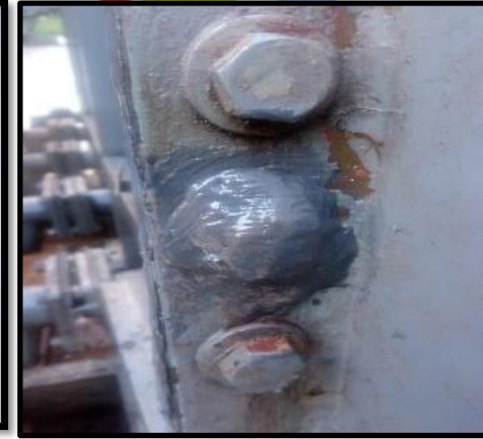
PTR Oil Leakage arrested in Saintala by Putty
