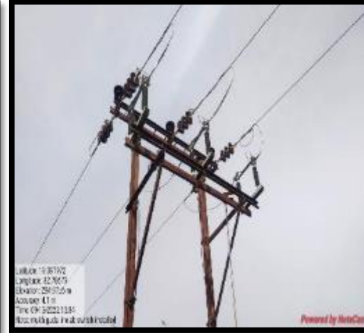
LINE AB SWITCH INSTALLED IN MUKHIGUDA PSS
