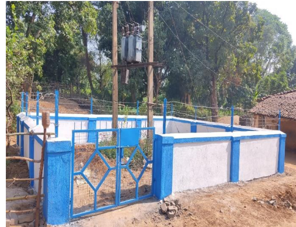
DTR fencing at Mundatikra, JED, under Sambalpur Circle
