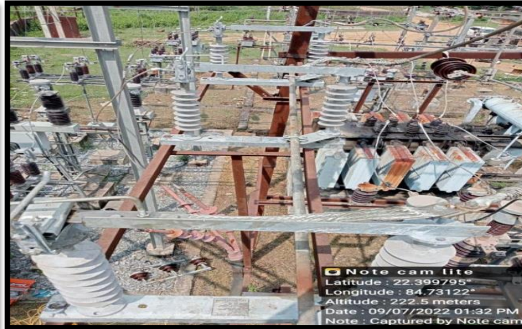
New 33KV AB Switch(400Amps) installed in 33KV BSL O/G Feeder at Biramitrapur PSS .
