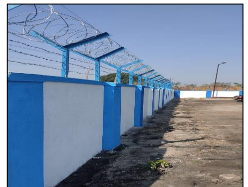
PSS Boundary wall work
