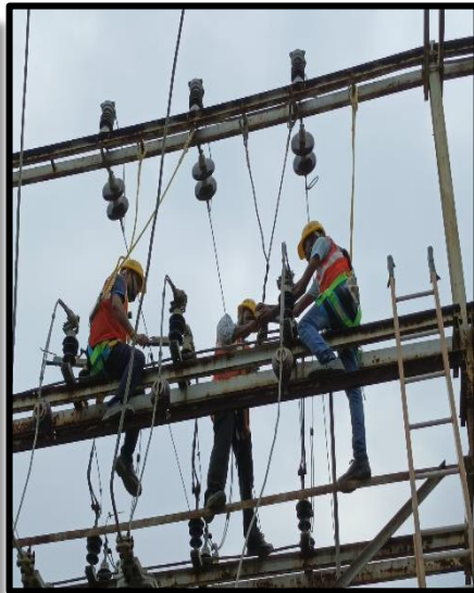
AB Switch Repairing WIP
