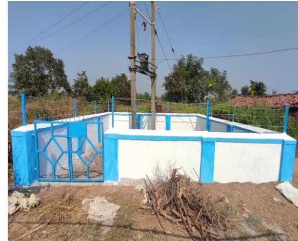
DTR fencing at Jiajhor, JED, under Sambalpur Circle
