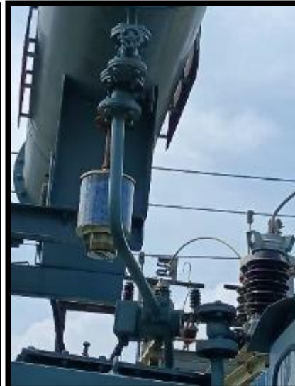
New 33KV AB Switch(400Amps) installed in 33KV BSL O/G Feeder at Biramitrapur PSS .
