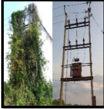
Project Clean up: Tree trimming & Preventive Maintenance
