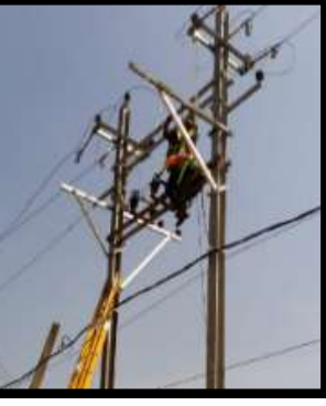
Priority Feeder Maintenance: LHGP, VoB & VoC feeder
