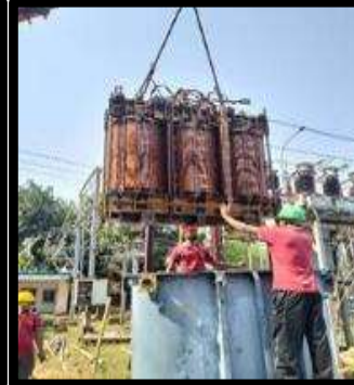
Project Navikaran: Onsite PTR overhauling – 45 Nos
