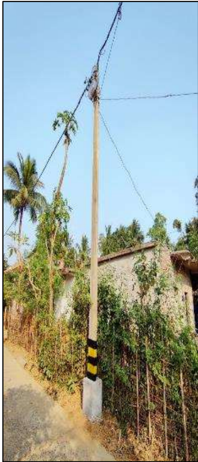
Service Cable Box
