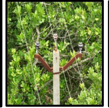
Drone Services: Feeder Audit, Thermo scanning – 26 feeders
