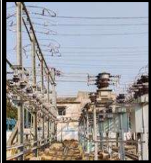
Circuit Breaker installation: VCB installed - 99
