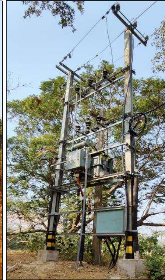
LT AB Cable Replacement
