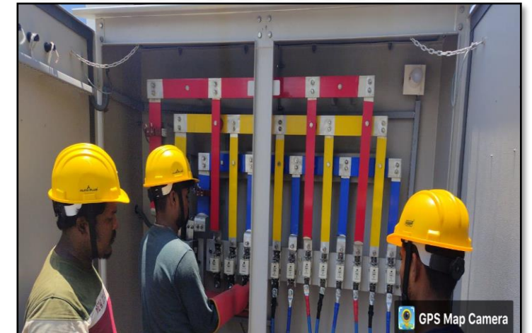
Installation of LV Protection at DSS
