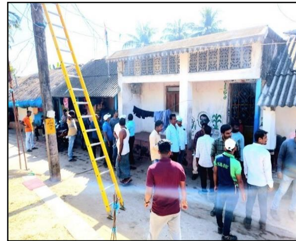
Friday Disconnection Drive
