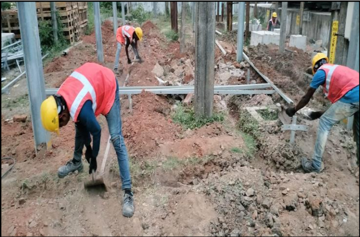
Earthing work at PSS
