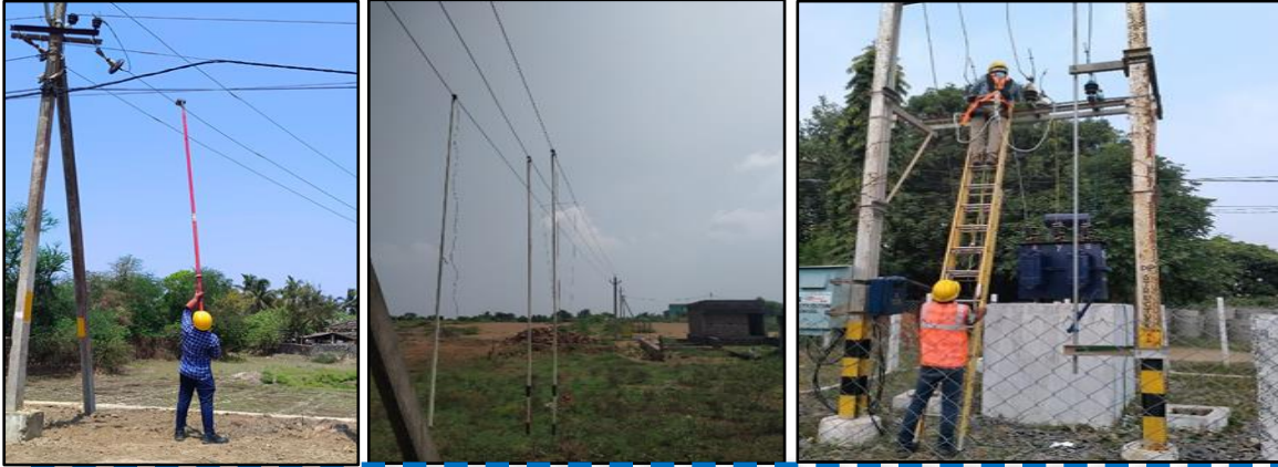
Deployment of Modern PPE & Safety Tools
