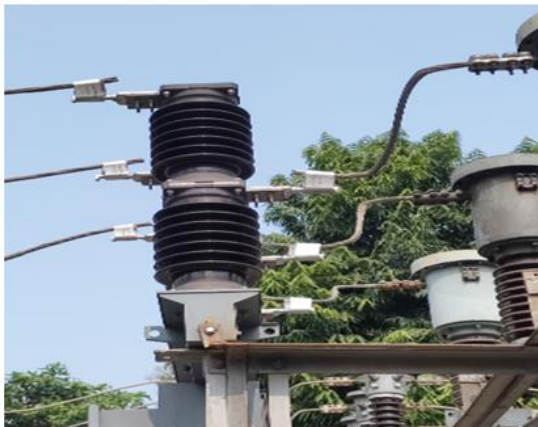
Installation of Wedge Connector
