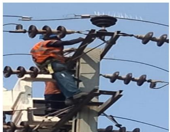
Installation of Bird Guard
