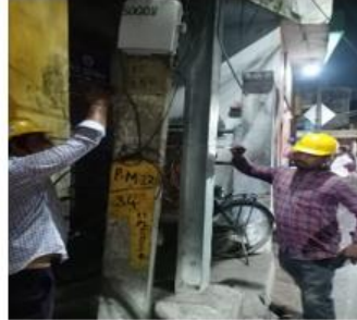
Leakage Current Testing of Poles
