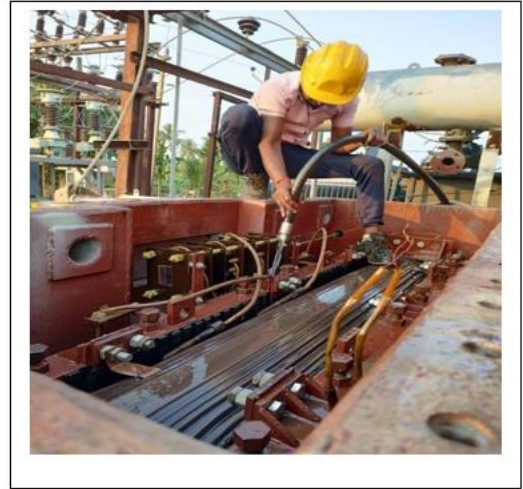
Refurbishment of PTR
