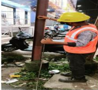
Leakage Current Testing of Poles
