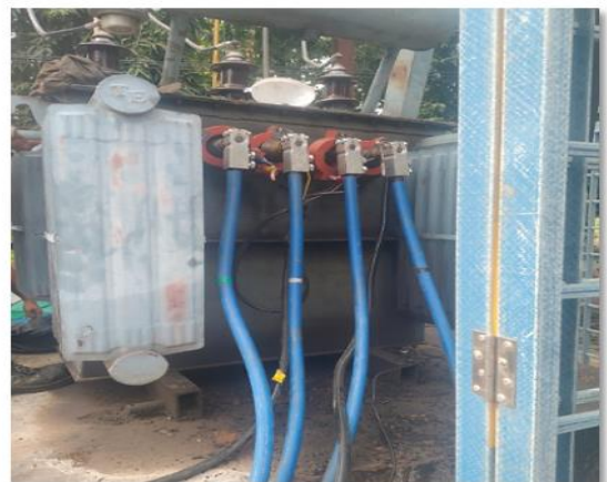
Installation of Bird Guard
