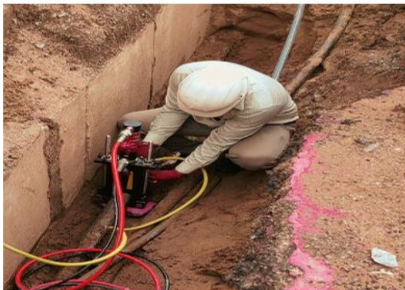
Cable spiking through Spiking Tool before cutting cable for jointing work
